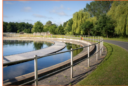
Heat from sewage
